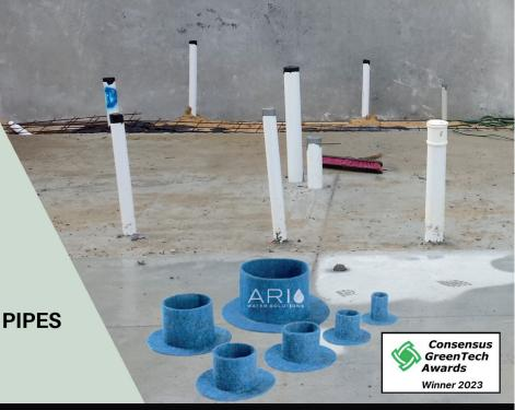
Easy to fit & cost effective way to prevent building waste entering DWV pipes whilst minimizing trip hazards.
